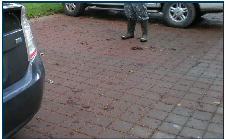
Native plants and pervious pavers were installed at Lake Sawyer for low impact access to the boat launch
