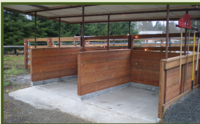
Waste Storage Facility
