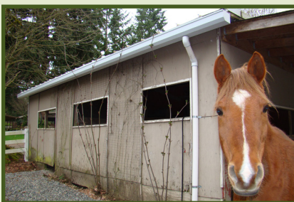
Roof Runoff Structure
