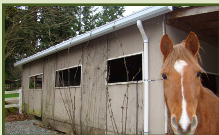
Roof Runoff Structure
